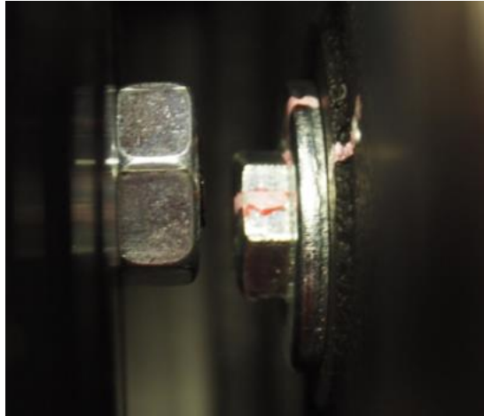
Figure 7. This auger pulley bolt (on the right side of the photo and marked with pink paint) is tightly secured against the pulley.
